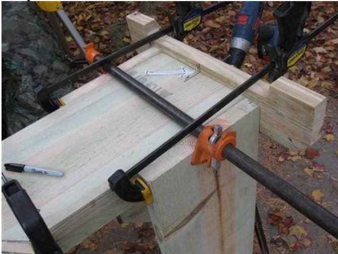
Repeat step two for all three remaining angled sideboards, using four screws each in the premarked holes.
